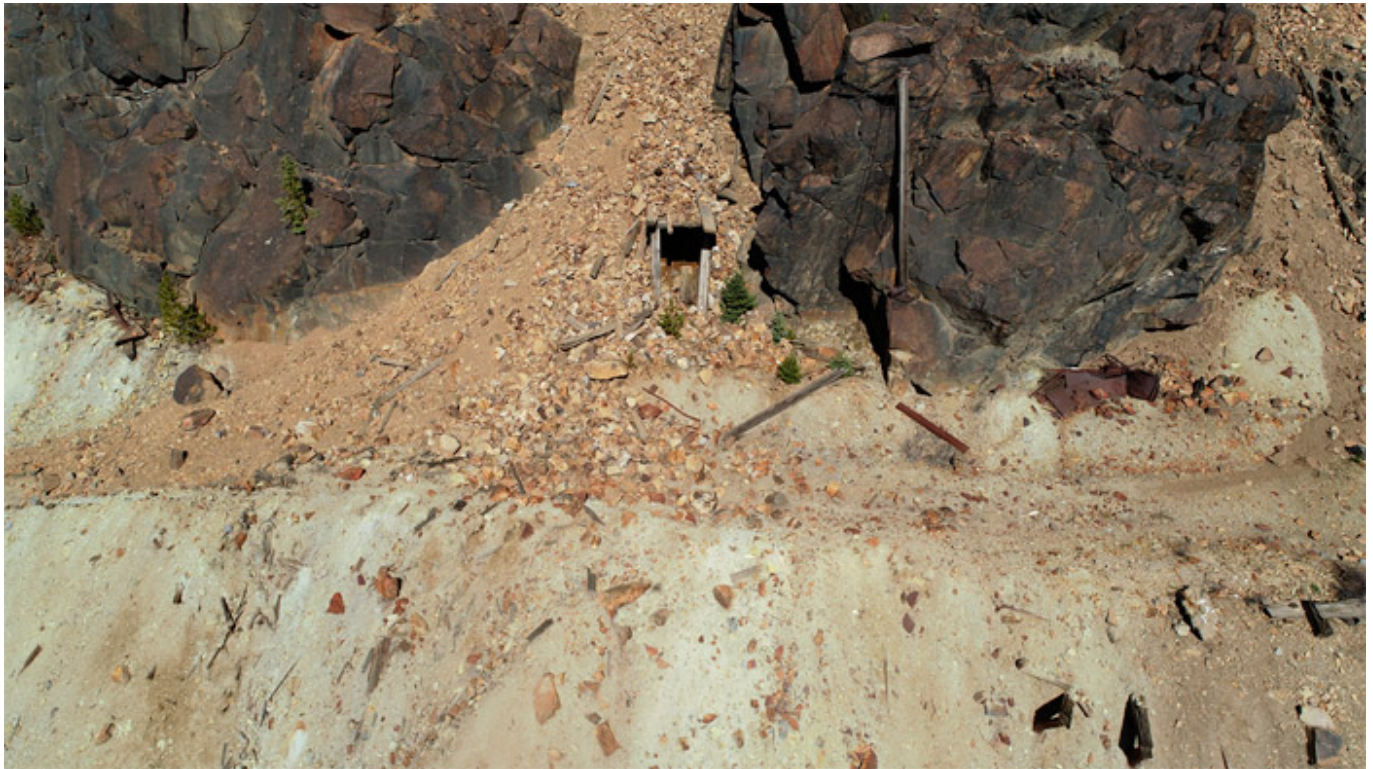
Figure 9-68. Mine opening only visible from oblique imagery.
