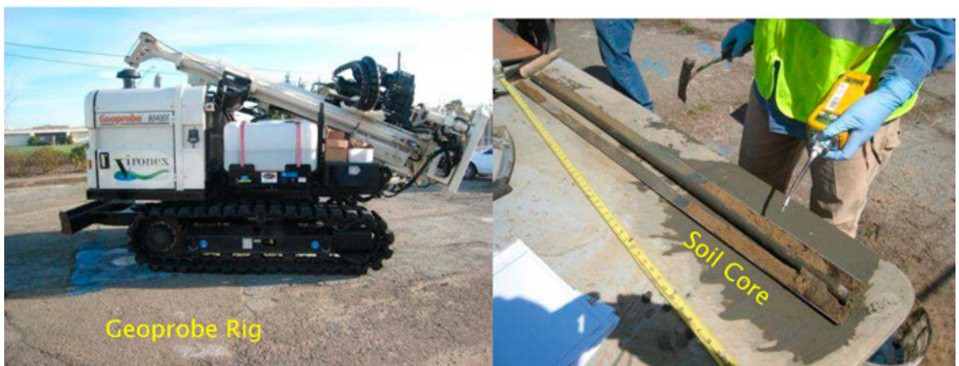
Figure 9-6. Soil core collection with Geoprobe DT8040.
